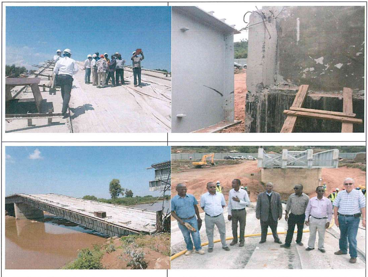
Investigations into collapse of Sigiri Bridge
